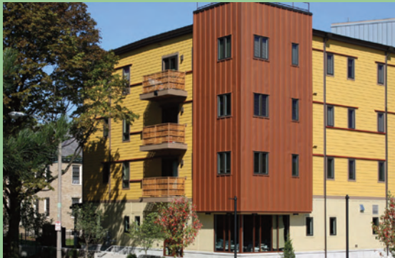
Saint Polycarp Apartments, Somerville, MA
