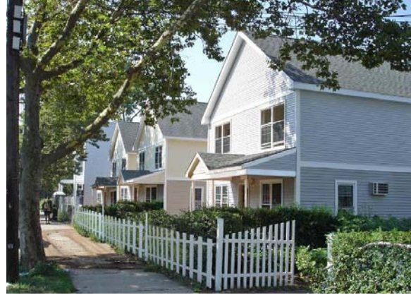
Ferry Street Mutual Housing
