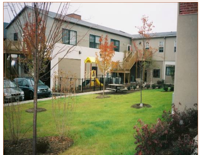
The New 401 Hazle Street in Tamaqua with 14 affordable apartments. Tamaqua Area Community Partnerships played a key role in securing this first NEF-financed LIHTC project for Rural LISC in Pennsylvania.
