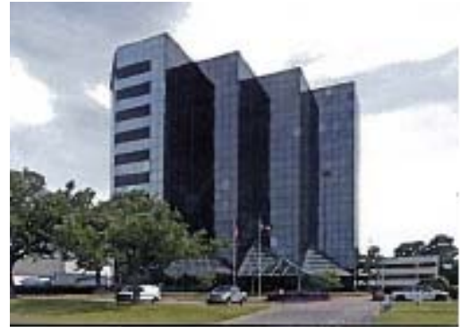
Park Central Plaza One 1111 North Loop West
