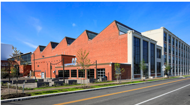
BELOW: Northland Workforce Training Center
