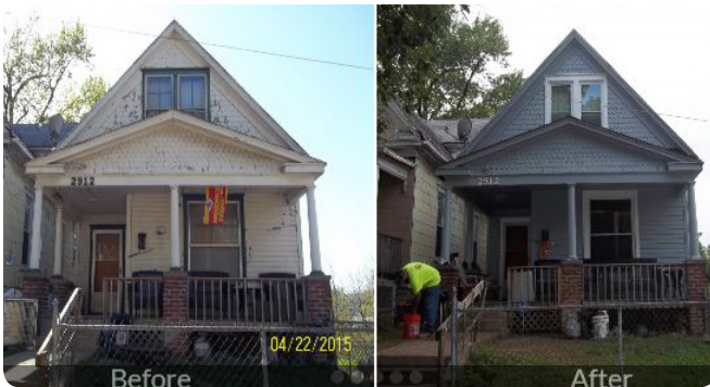
Before and after images of a WHO home repair project.
