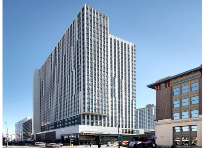
The Crossing at Jamaica Station Jamaica (Queens), NY completed 2020 Development Total Development cost $405,000,000
