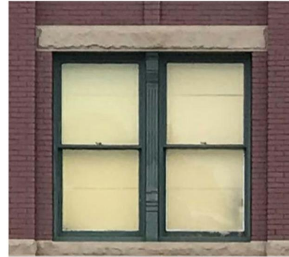
SYNDICATE BLOCK - EXISTING 2ND FLOOR WINDOWS
