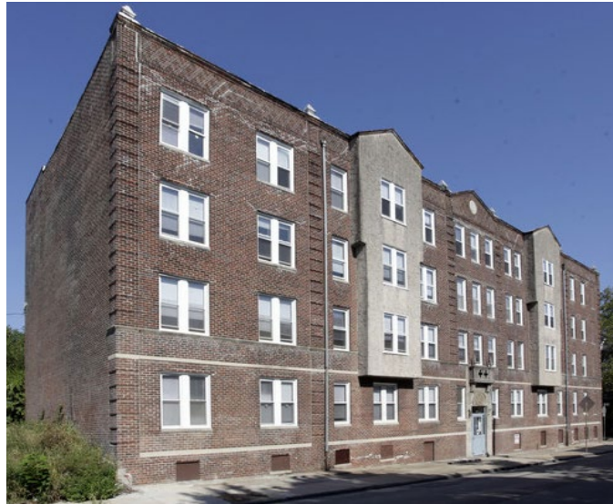
Tioga Arms Apartments in North Philadelphia
