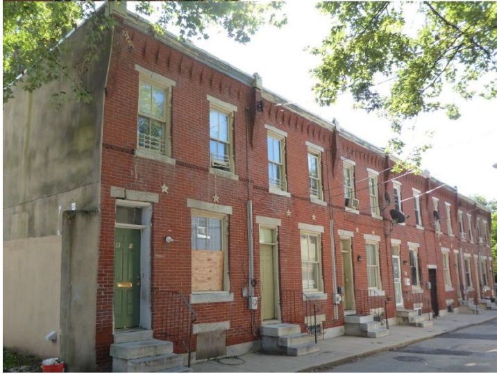
FRP Community Homes in West Philadelphia
