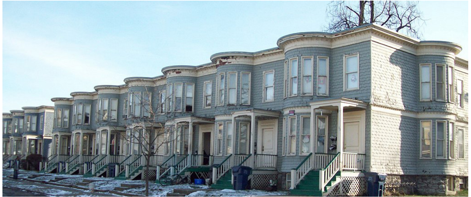
Emerson Place Rowhouses. Photo: Buffalo Commons Photobank
