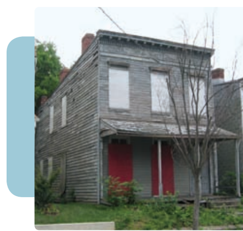
"RIBBON HOUSE" before renovation
