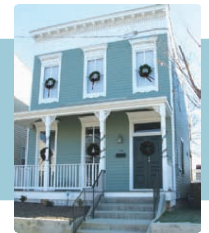
"RIBBON HOUSE" after renovation
