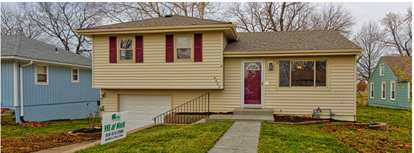
Photo of a Northland home after Home Repair. Courtesy of Northland Neighborhood, Inc.
