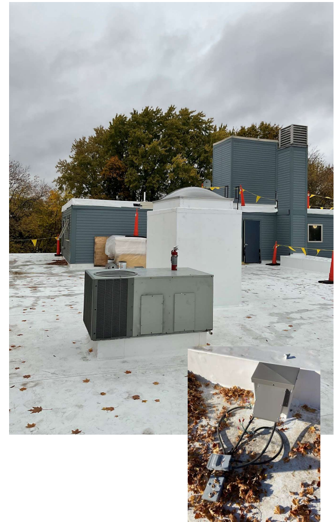
New TPO Roof being installed
