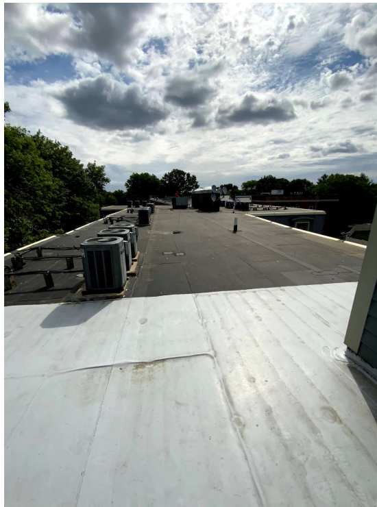
Building orientation excellent for solar array
