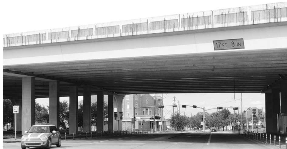
Photo of Intersection between US 59/I69 and Lyons Avenue
