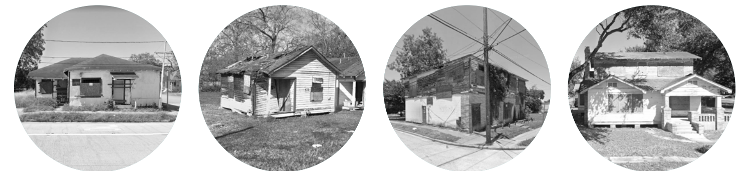
Examples of "Unsound" Residential Structures
