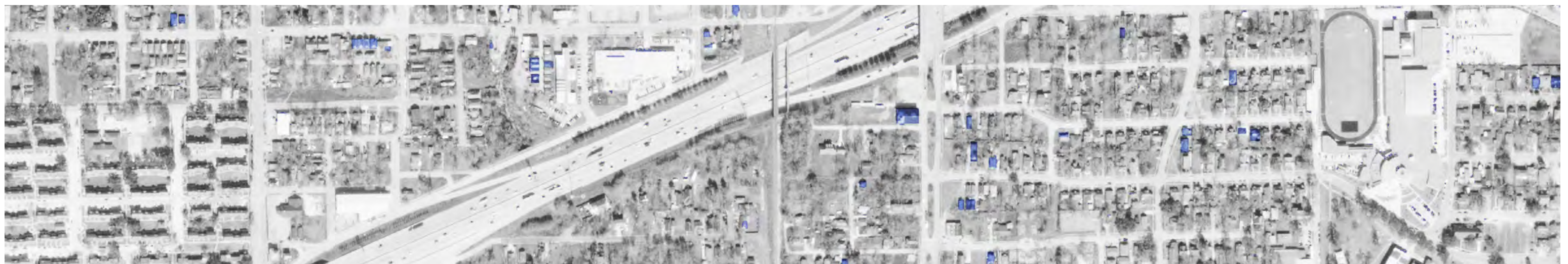
Aerial Highlighting Blue Tarp Roof Tops after Hurricane Ike in 2008
