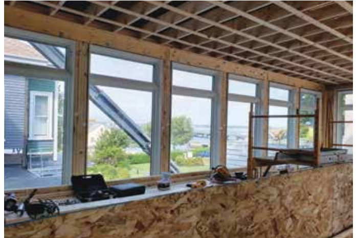
A rehab on 38 apartments for seniors, Newport, RI
