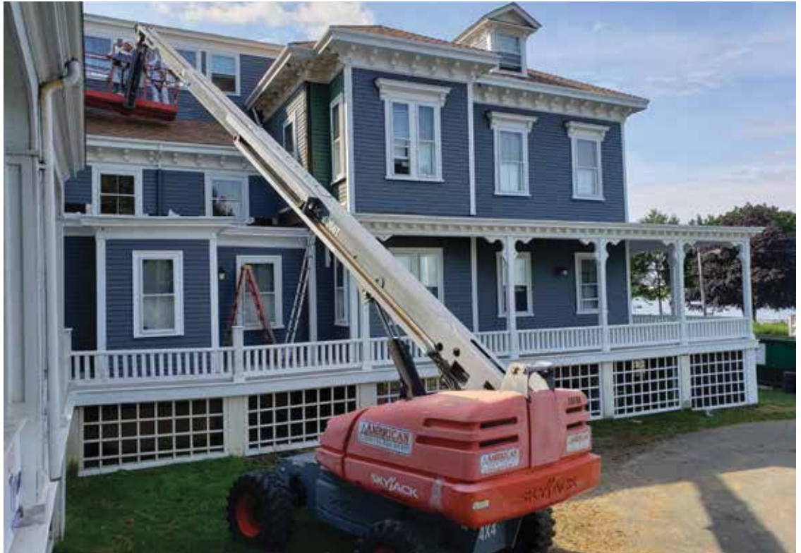
Harbor House Senior Housing, Newport, RI
