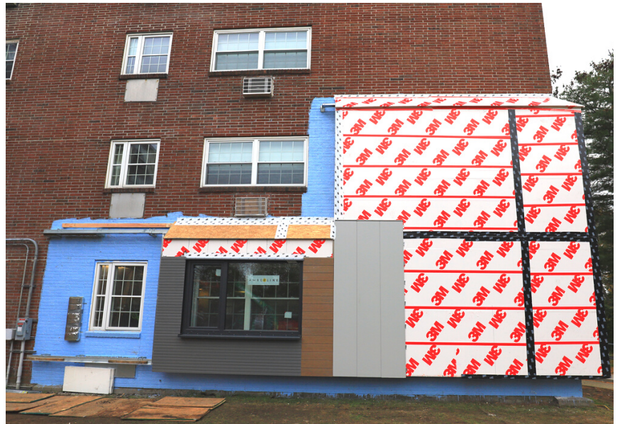
Fairweather Apartments, Salem, during a panel installation demonstration, prior to starting construction.
