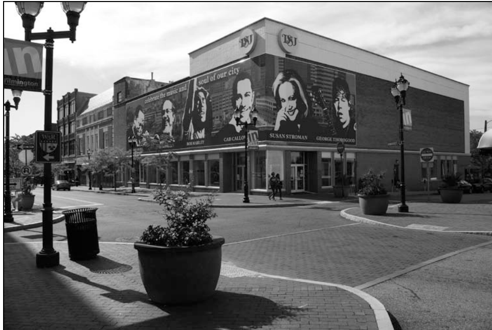
Figure 2.16 Streetscape improvements at Seventh and Market Street (photograph by author, taken October 17, 2010)
