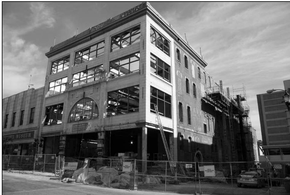
Figure 3.10 Queen Theater during restoration ( photograph by author, taken October 17, 2010 )
