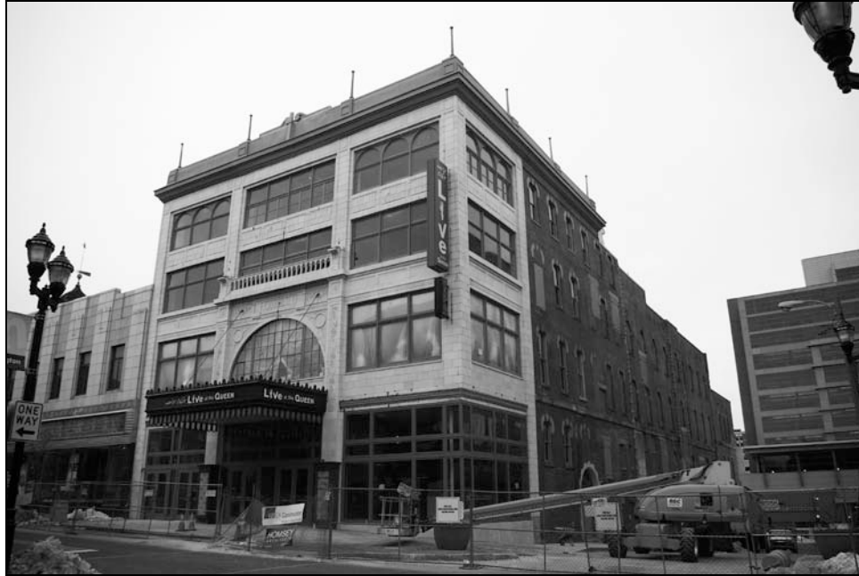
Figure 3.11 Queen Theater nearing completion ( photograph by author, taken February 8, 2011 )
