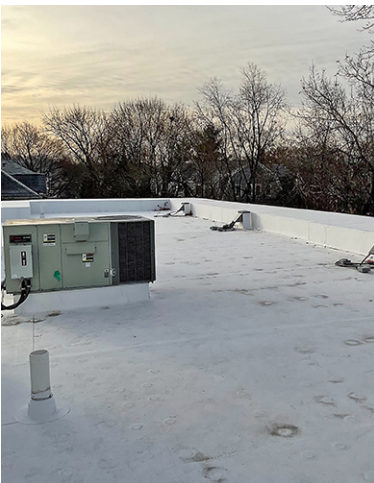
Above: A full roof replacement was needed, including insulating to R-50. Below: Installation of a white roof membrane in preparation of a future solar PV system.
