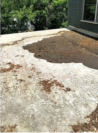
Above: A full roof replacement was needed, including insulating to R-50. Below: Installation of a white roof membrane in preparation of a future solar PV system.
