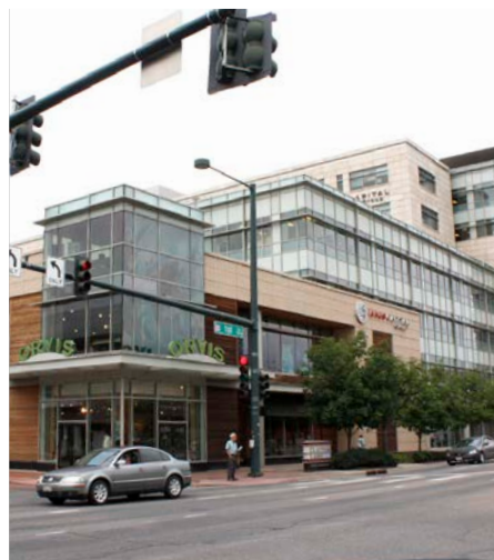
SCALE TRANSITIONS The interstate fronting development should transition to that of the 3 story neighborhood.
