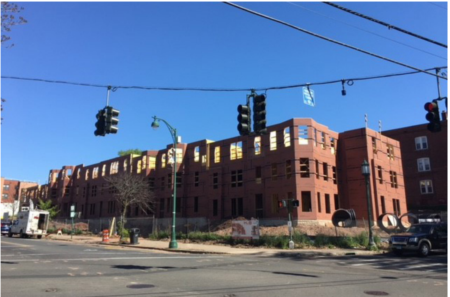
MHAGH: HUB on Park, 36 units under construction (now complete)
