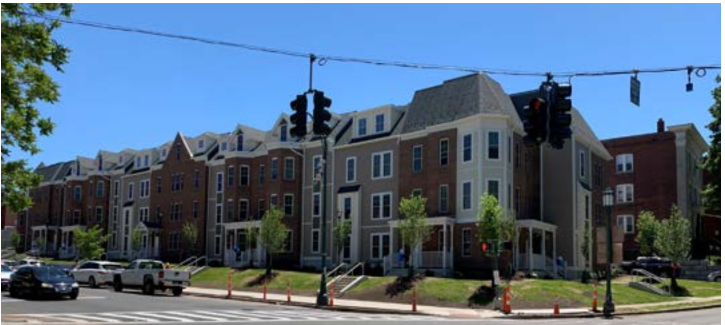
MHAGH: HUB on Park St, 36 newly constructed units
