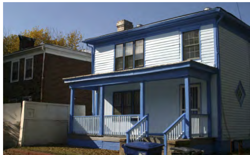
(ABOVE) Photos showing the character of rehabilitated housing in the Rome Street neighborhood
