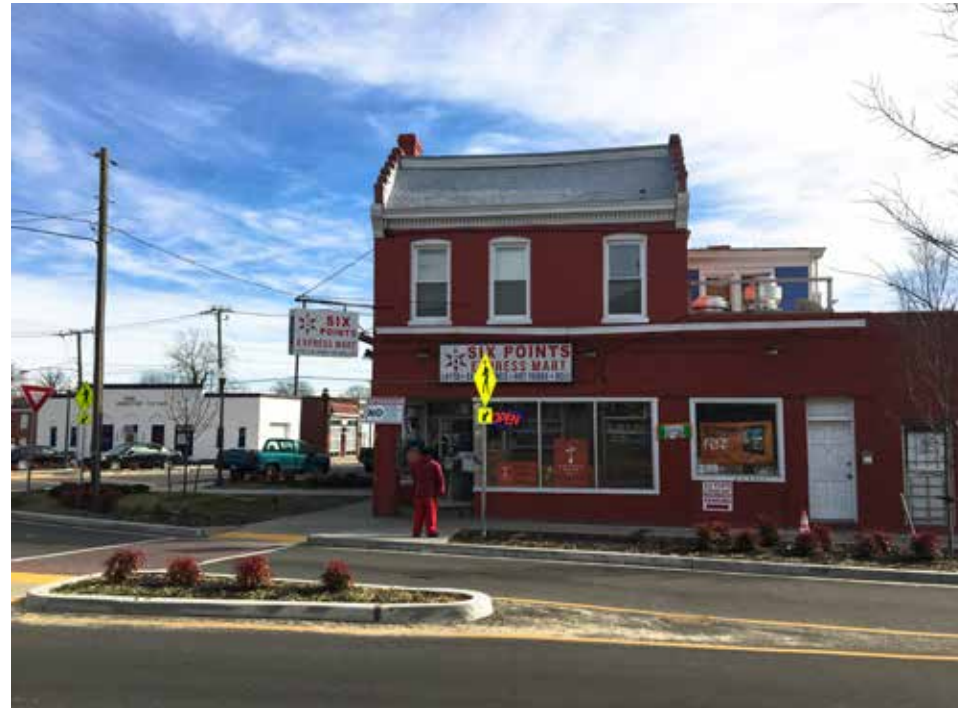
The roundabout at Six Points includes curb bump-outs, pedestrian islands, and new crosswalks that make the area safer and more comfortable for pedestrians and a more desirable destination for local residents and customers.
